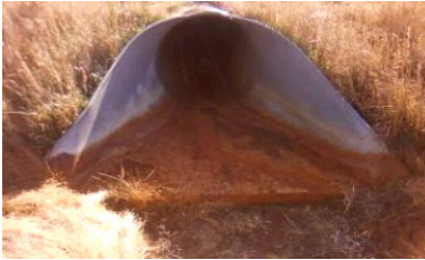
Moderate: Rust or scaling with minor section loss
