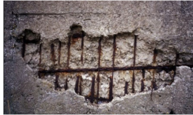
Moderate: Rust or scaling with minor section loss
