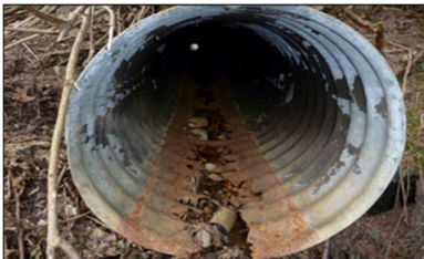
Severe: Complete material section loss (holes)
