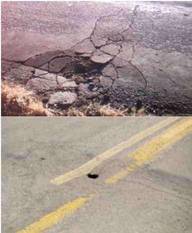
Common Culvert-Related Road Surface Distresses
