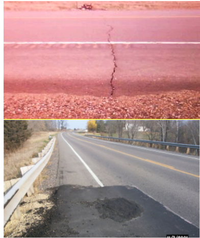
Common Culvert-Related Road Surface Distresses
